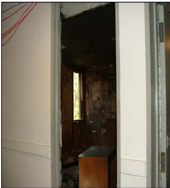
Corridor outside the room
