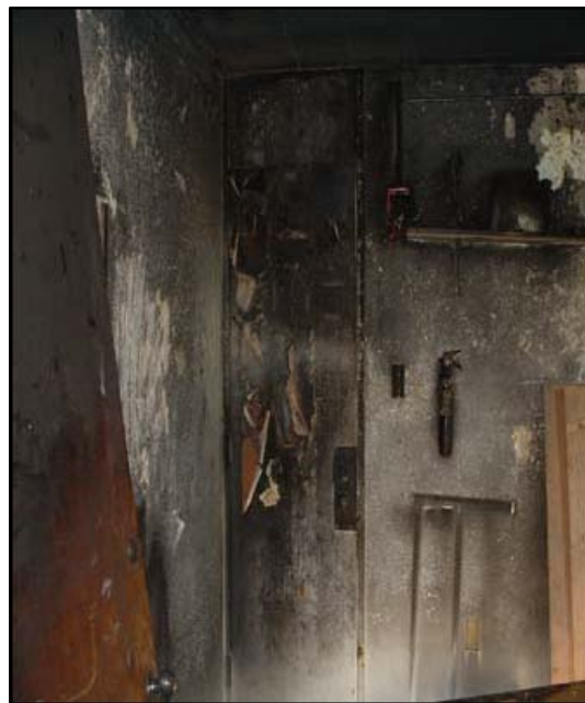
Interior of the room
